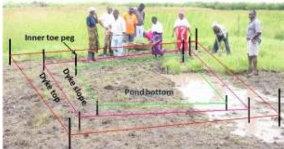
4: A site pegged ready for digging and filling (Mbugua H. M.)
