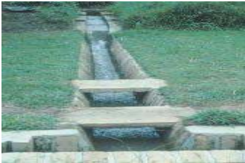
15: An open water supply canal lined with concrete slabs (Ngugi C. N.)
