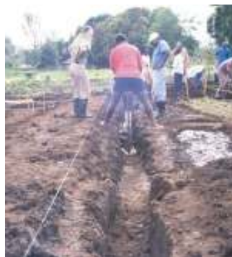
9: Fill the trench with moist clay and compact thoroughly (Ngugi C. N.)
