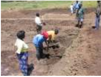
10: Shape the dyke slope and the pond bottom (Mbugua H. M.)
