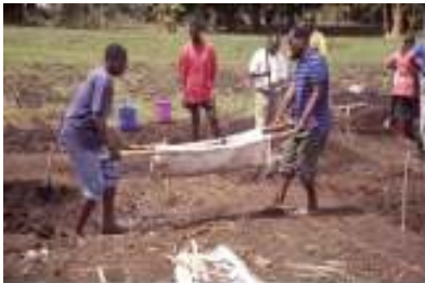
13: Soil can be moved using simple locally assembled equipment e.g. a stretcher made of sticks and old gunny bags locally known as 'machela'. (Ngugi C. N.)
