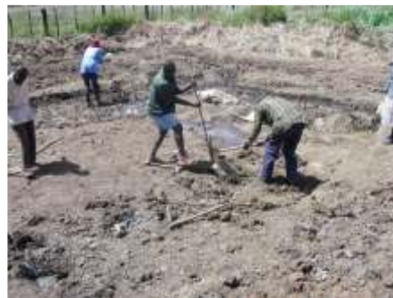
6: Make sure that you remove all boulders and tree stumps from the pond area (Mbugua H. M.)
