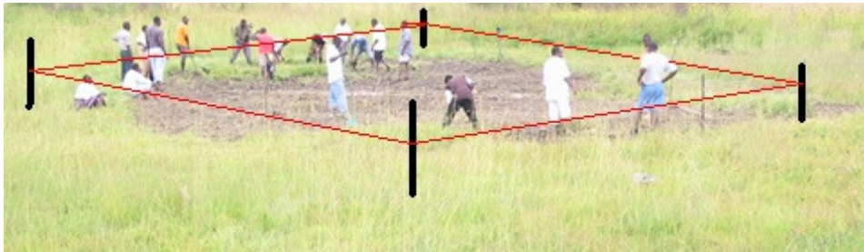
Figure 3: Clearing vegetation from the pond site (Mbugua H. M.)
