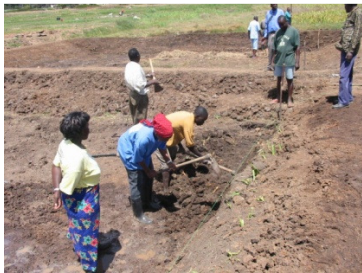
10: Shape the dyke slope and the pond bottom (Mbugua H. M.)
